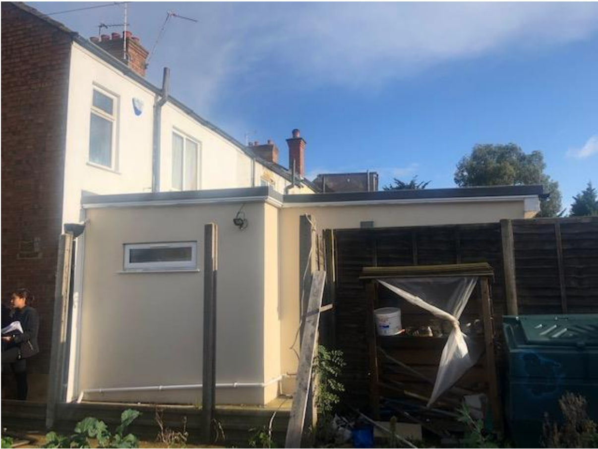
View of No. 15 Kingsley Road
