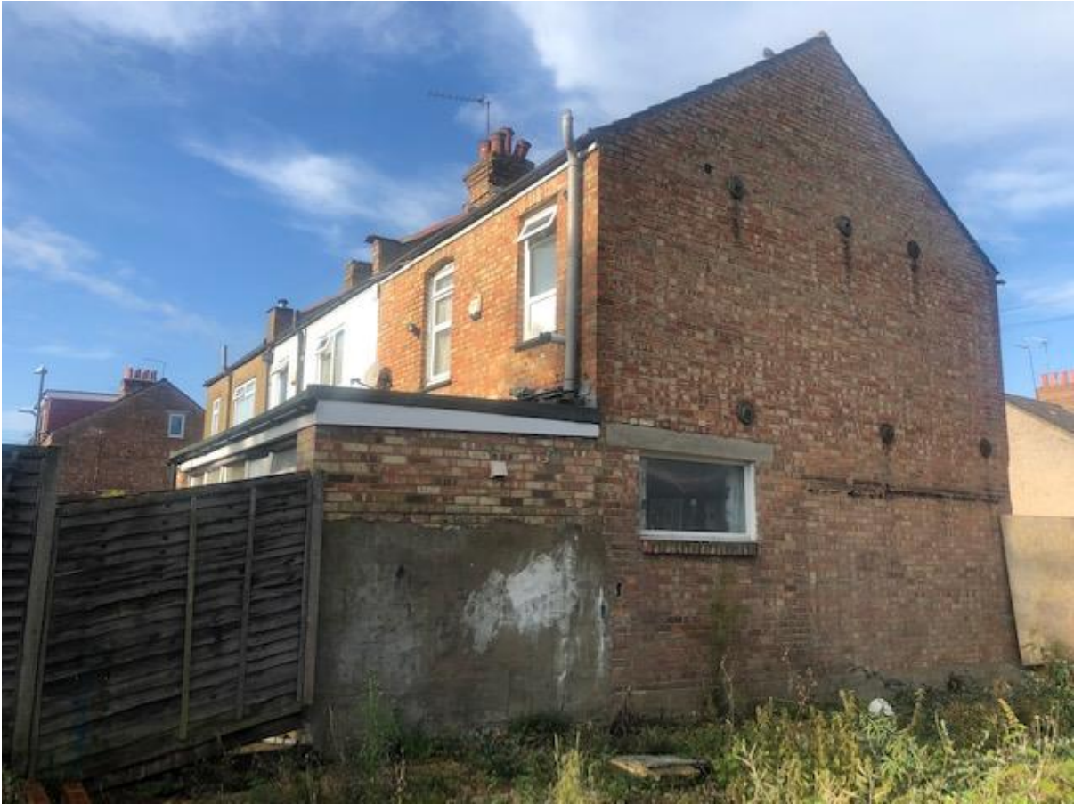
View of No. 23 Kingsley Road
